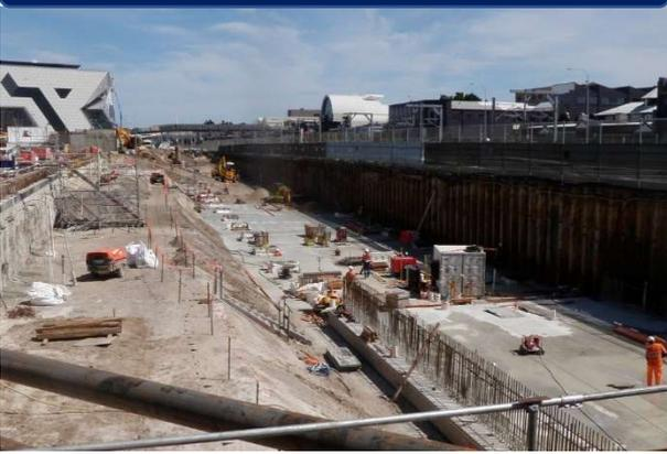
The Perth City Link project consists of “sinking” the rail line and the Wellington Bus Station to create a 13.5 hectare space that will be used for housing and business.
